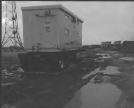
Wind-Diesel Battery Hybrid for Kwigillingok
