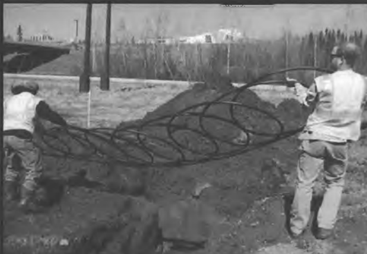
Installation of Slinky Loop
