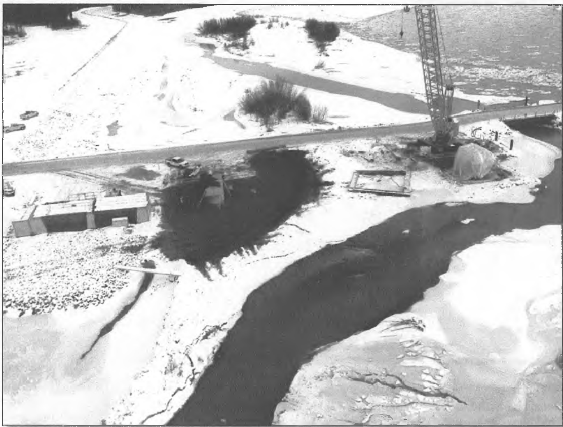
Above: Piers 3 and 4 under plastic tents during construction to keep inside environment warm. Below: Pier 2, the first completed pier.
