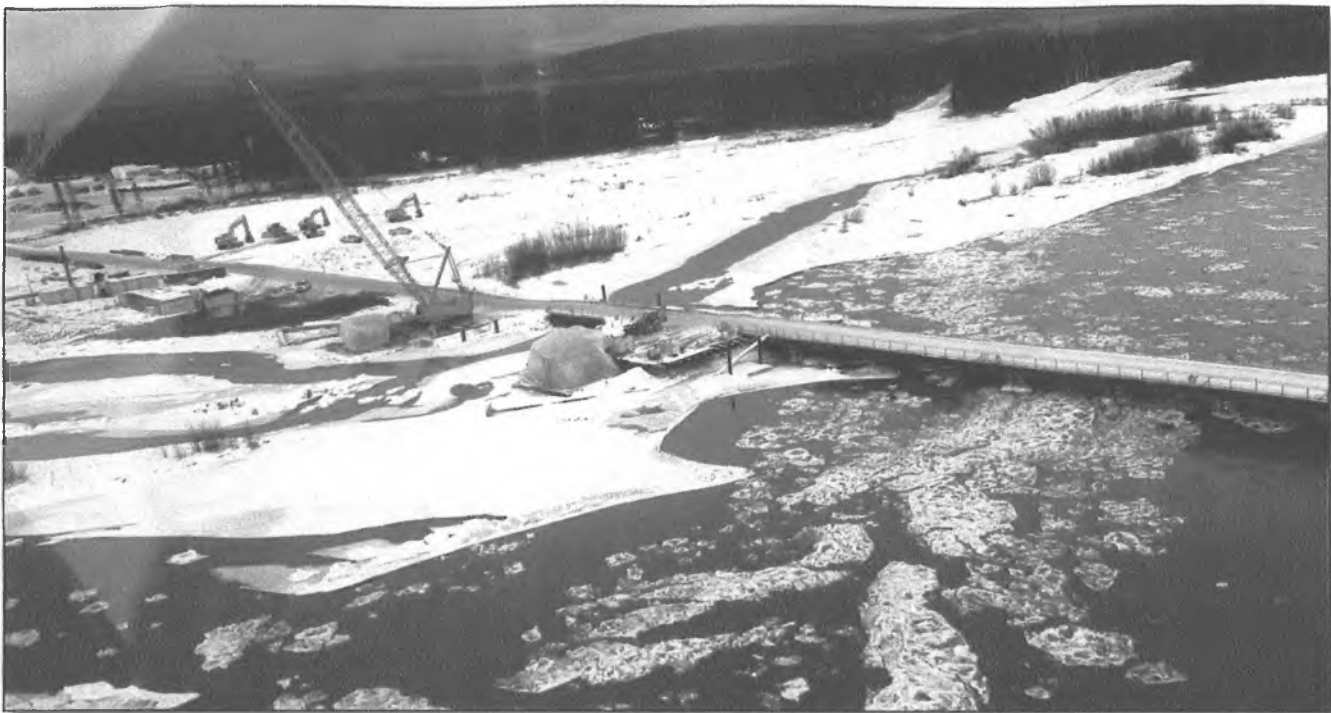
Above: Piers 3 and 4 under plastic tents during construction to keep inside environment warm. Below: Pier 2, the first completed pier.
