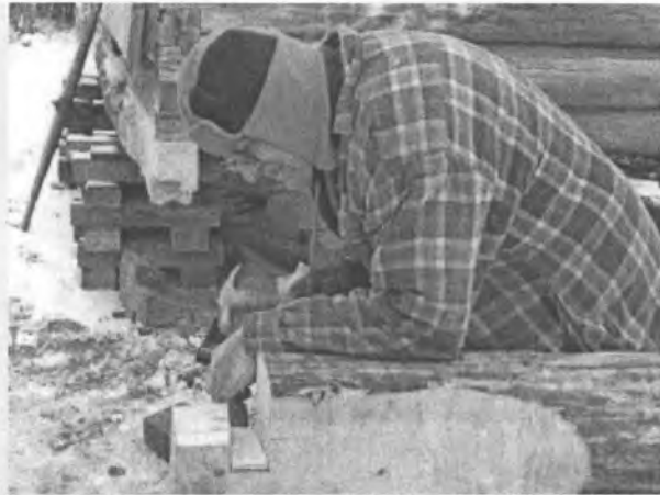
Photo courtesy of Gary Titus. Mike Wiley employs a hammer and chisel to fashion a step-and-lock notch that will fit up into the similarly notched sill log in the background on the historic Watchman’s Cabin in Kasilof.
