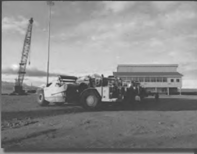
Barge dock staging area
