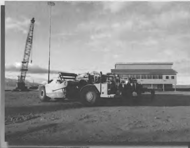
Barge dock staging area
