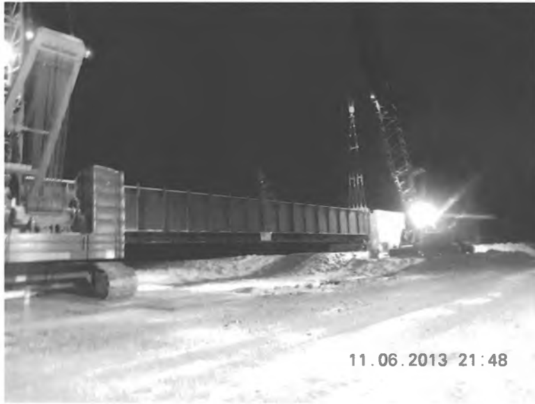
Last bridge girder erected
