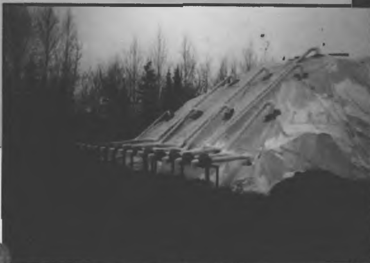
Contaminated soil is aerated as part of some treatment processes.
