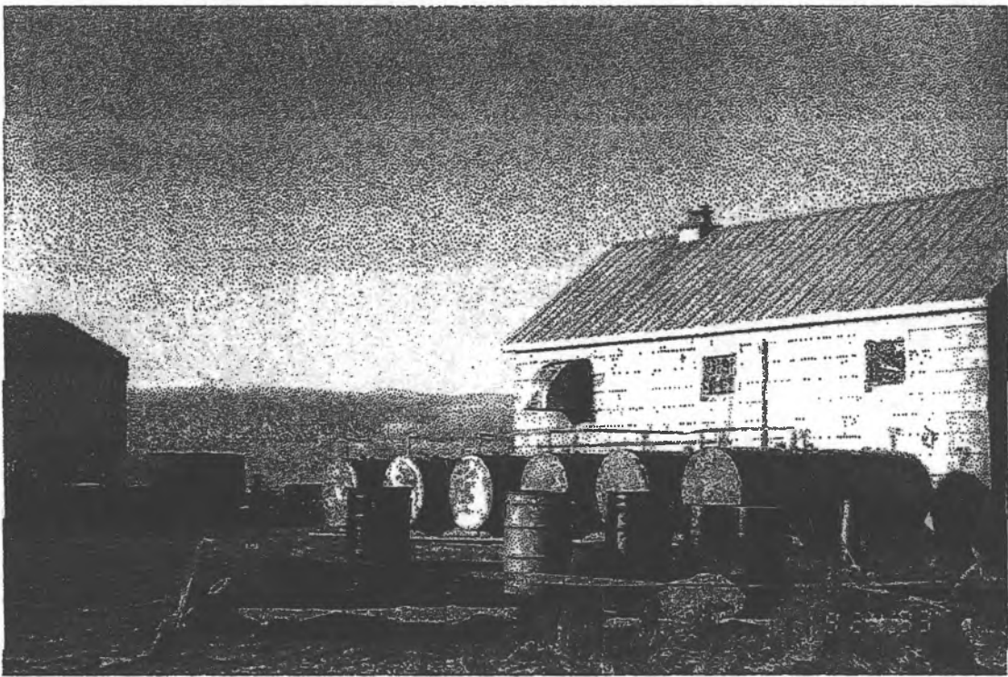
Figure 5. Tank Farm/Power Generation Building at Middleton Island
