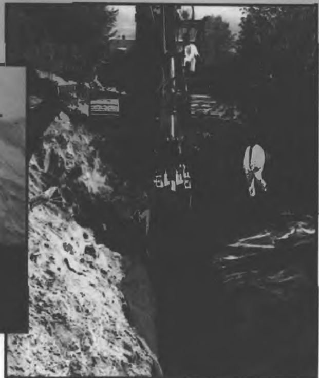
A lined trench intercepts contaminated substances during a major site cleanup.
