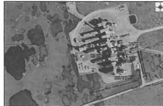
PBU Central Gas Facility Tie-in
