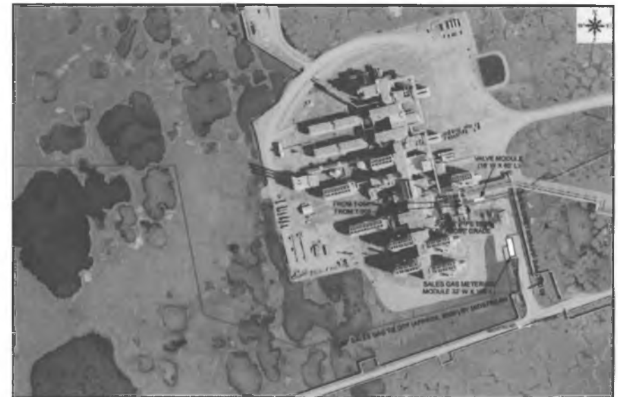
PBU Central Gas Facility Tie-in
