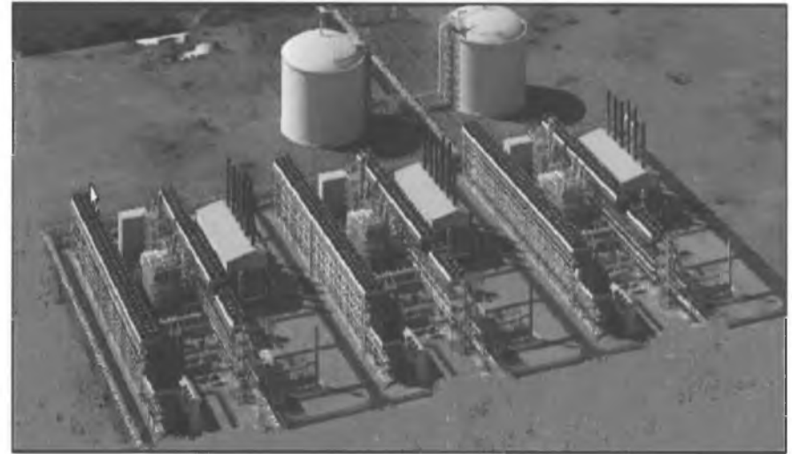
SCLNG Plant and Storage
