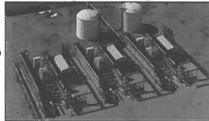
SCLNG Plant and Storage
