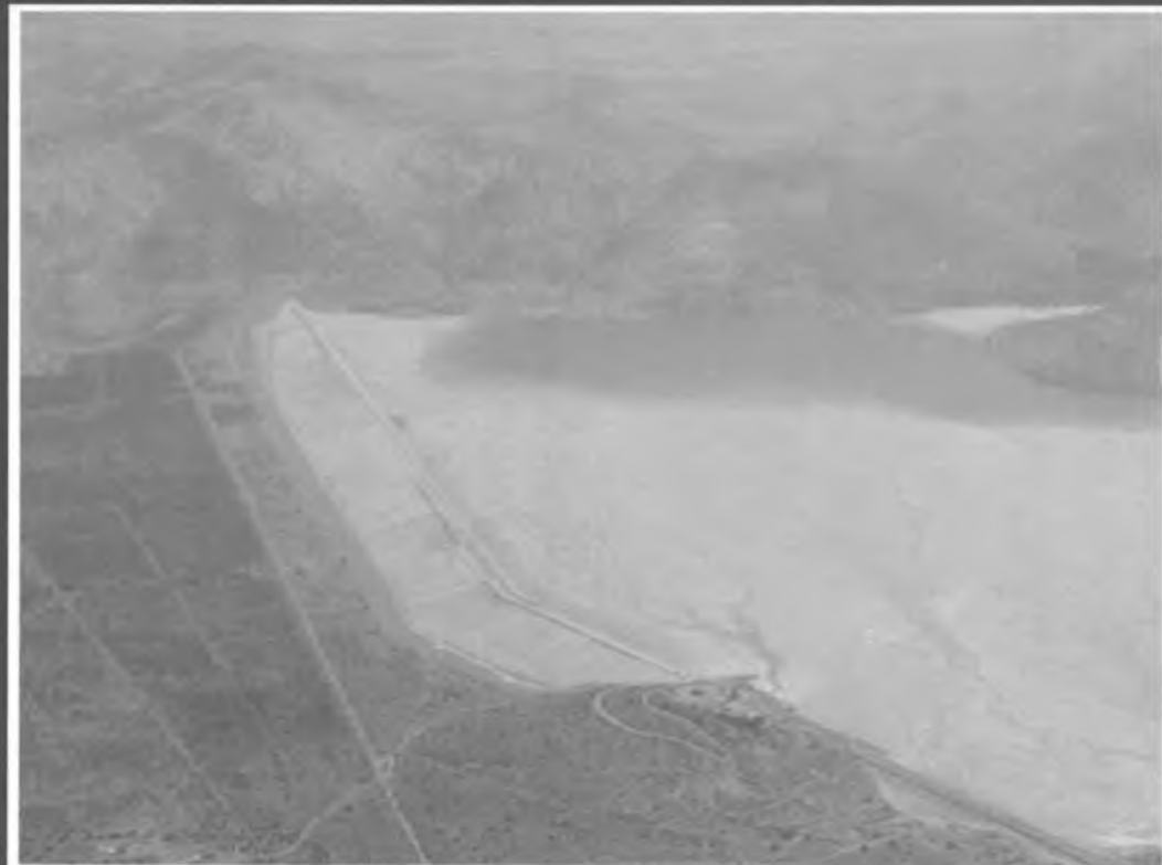
Figure 11.8. March 10, 2010 View of Ovejera Tailings Dam from Helicopter (S33.054182°, W70.768953°)
