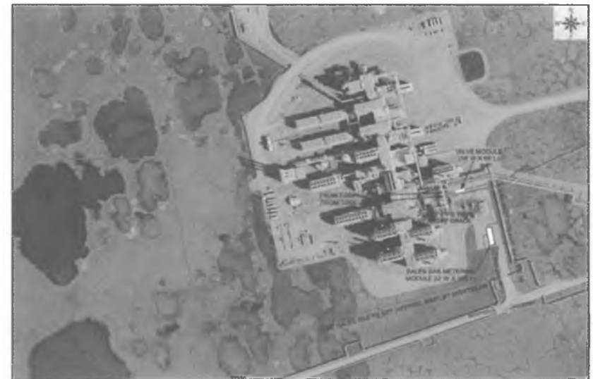
PBU Central Gas Facility Tie-in
