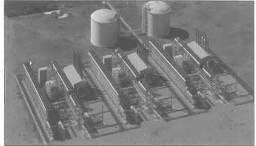
SCLNG Plant and Storage
