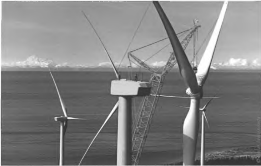
CIRI's Fire Island Wind turbines
