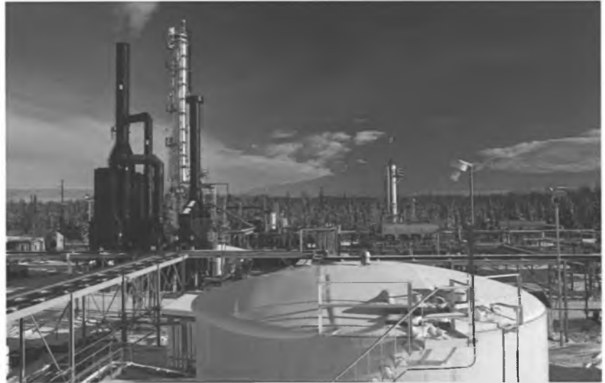
Petro Star refinery at the North Pole
