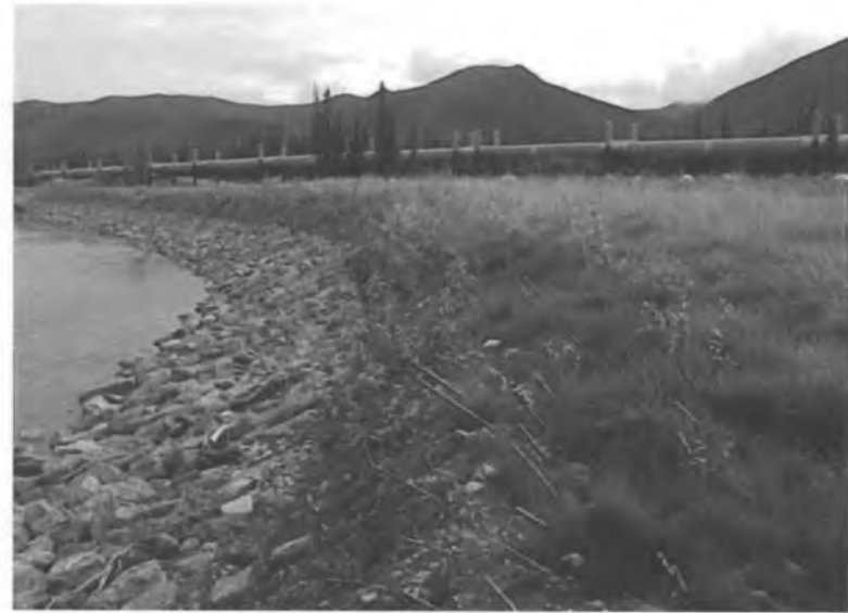
Stream revetment and pipeline
