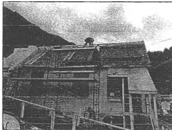
New roof on the St. Nicholas rectory
