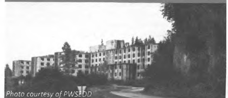
Buckner Building, Whittier
