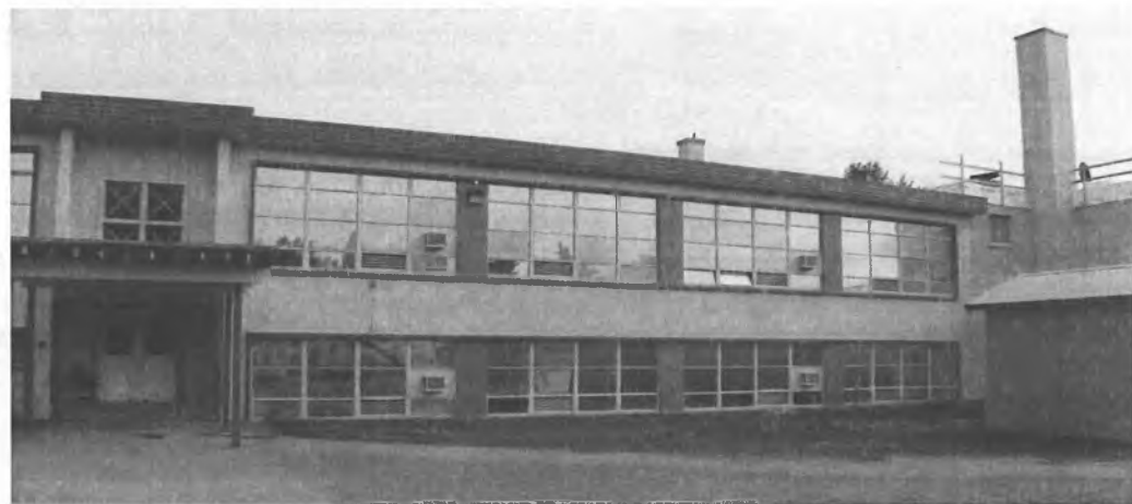
Figure 1: View of South Facing Windows with A-C Units
