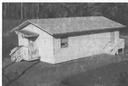
Figure 1: View of Chinook Elementary Relocatable Classroom
