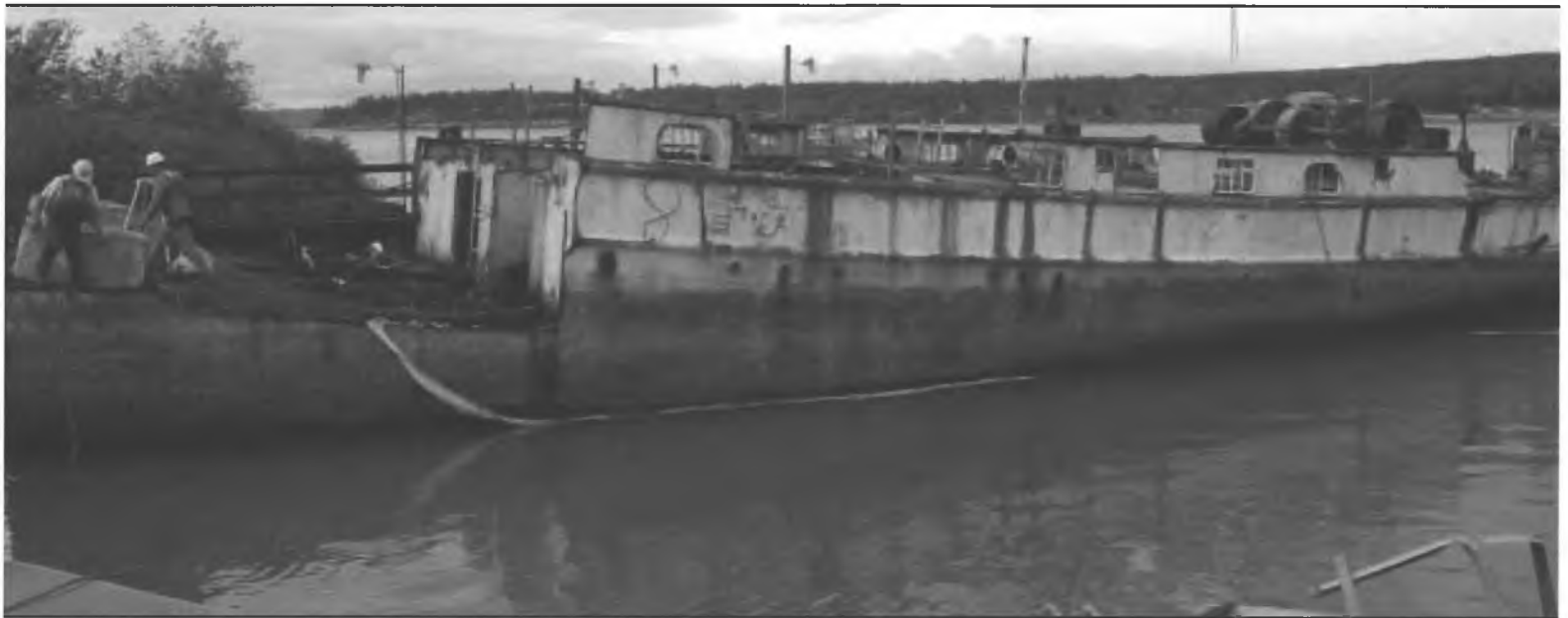
A derelict vessel is dismantled on a bank of the Snohomish River in Everett, Wash. U.S. Coast Guard photo by Chief Petty Officer Paul Roszkowski.
