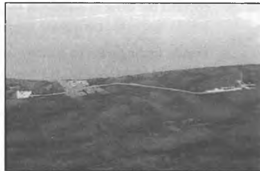
This aerial view of Mertarvik shows the significant progress made to date, June 2011. Photo by Harvey Smith.
