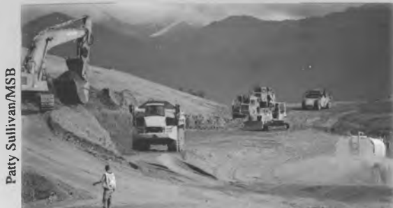
Photos: the ship, the deepest draft vessel ever in Upper Cook Inlet at Port MacKenzie; Above: 2010 haul road and rail loop construction at Port Mac moved 1.9 million cubic yards of dirt.
