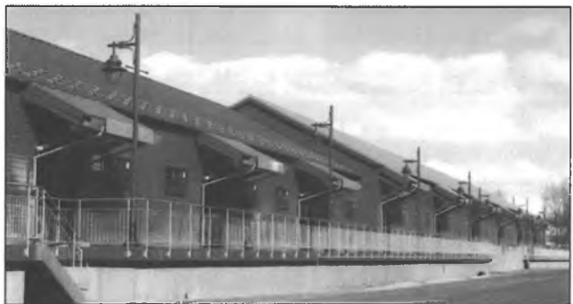
The Historic Freight Shed renovation nears completion.
