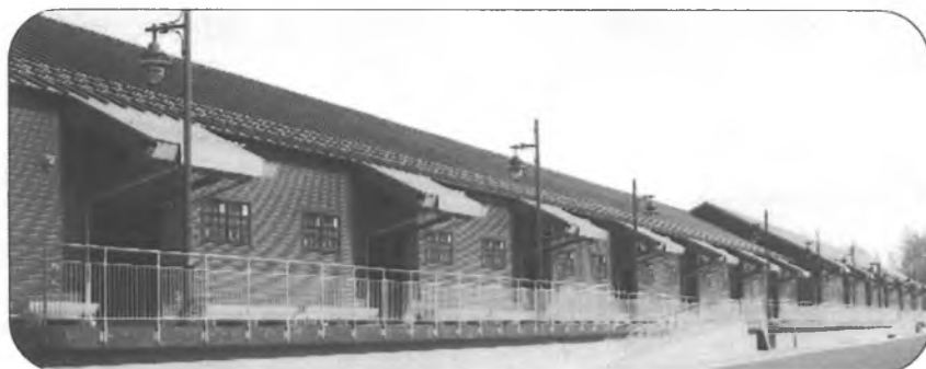
RENOVATING THE HISTORIC FREIGHT SHED TO LEADERSHIP ENERGY & ENVIRONMENTAL DESIGN (LEED) STANDARDS IS A MAJOR INTERNALLY-FUNDED PROJECT.
