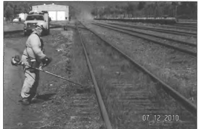
Ineffective mechanical/manual control in Seward yard prior to herbicide application.
