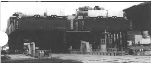
The Whittier barge slip stern (front) is replaced. The towers were removed and replaced by hydraulic devices to lower/raise the slip.
