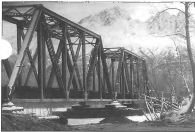
Matanuska River Bridge is undergoing rehabilitation work.
