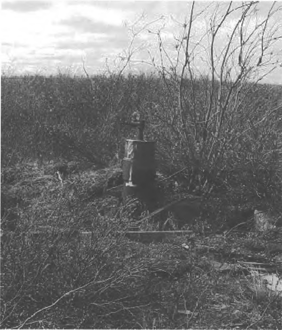
Primitive, rusting wellhead and wood debris
