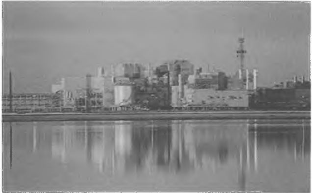
Lisburne Processing Center
