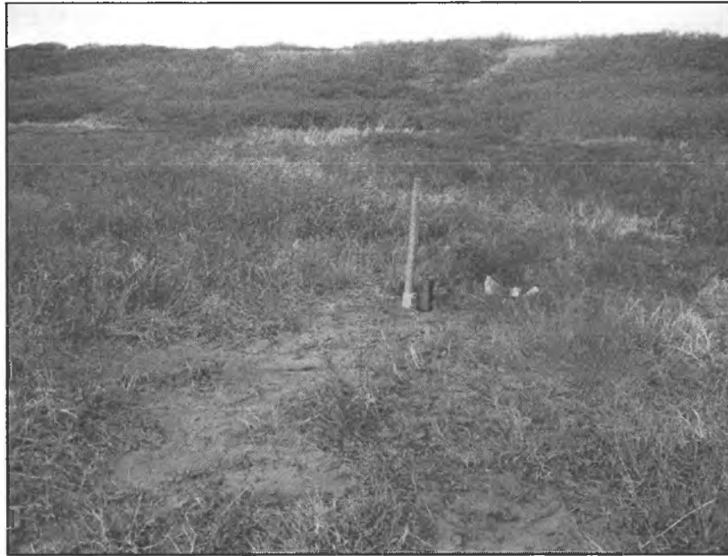
After drill removed
