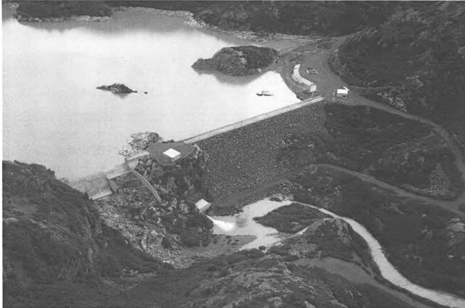
Example of embankment dam
