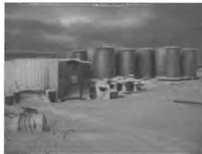
Rural Alaska fuel storage tanks
