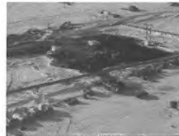
Leak and spill
