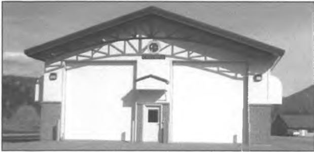
The prototype section maintenance facility built in Cantwell.
