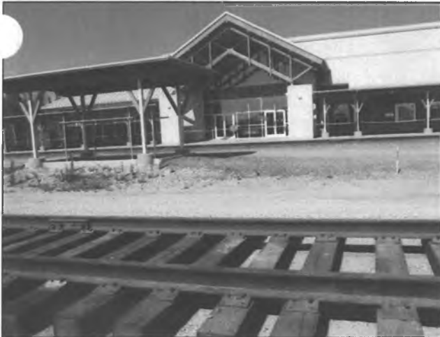
A second track is constructed parallel to the existing track by the Fairbanks Depot.
