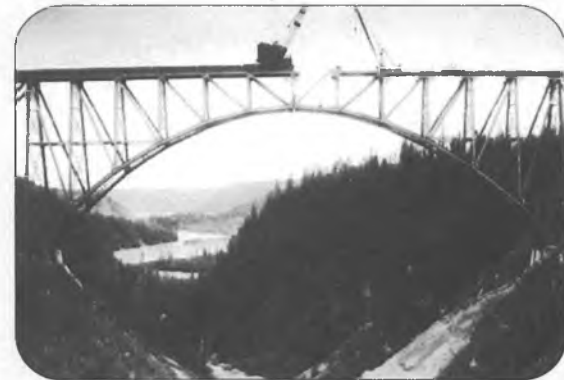
HURRICANE BRIDGE UNDER CONSTRUCTION. CIRCA 1921.
