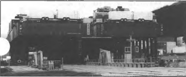
The Whittier barge slip stern (front) is replaced. The towers were removed and replaced by hydraulic devices to lower/raise the slip.
