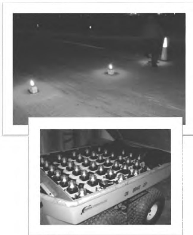
On a clear night lights are visible 5 miles out on approach to the airport. Emergency runway lights are easily stored and installed.
