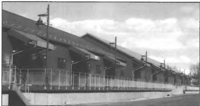
The Historic Freight Shed renovation nears completion.
