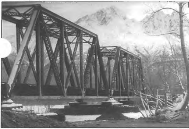
Matanuska River Bridge is undergoing rehabilitation work.
