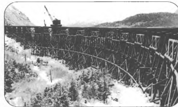
BRACE WORK TO STIFFEN THE LOOP DISTRICT TRESTLE AT MILE 48.3. CIRCA 1948.
