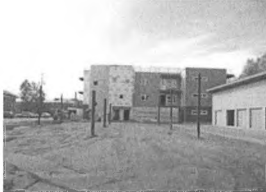
Photograph of Property (construction underway):
