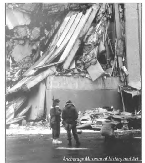
The J.C. Penny building in downtown Anchorage was heavily damaged during the 1964 Good Friday earthquake.
