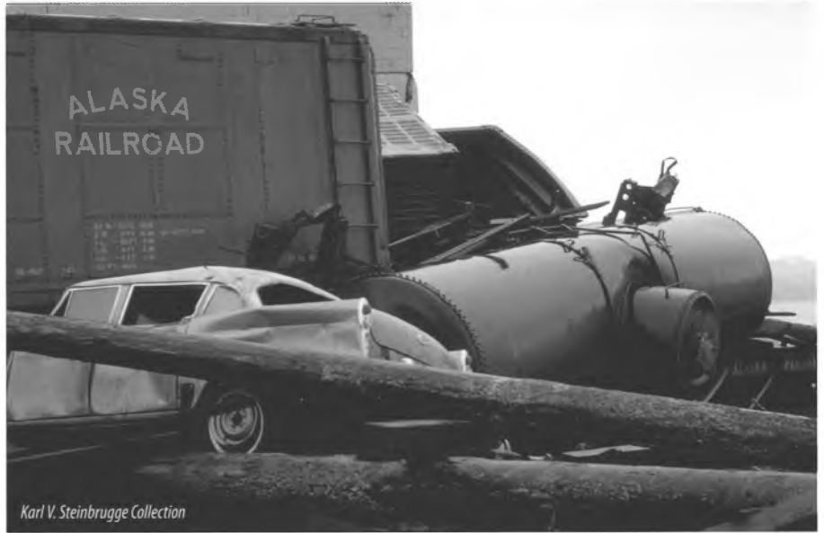
Damage in Seward following the 1964 earthquake. The waterfront area, railroad yard, and petroleum storage tank facilities were devastated by the tsunami.
