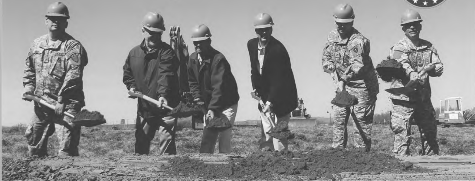
New Bethel Readiness Center Begins. The official party digs up dirt as a sign of “breaking ground” for the start of construction of the new Bethel Readiness Center. So far, the contractor has poured the concrete, insulated side panels and put roof panels in place. The project is ahead of schedule and is expected to be completed by December 2011. From left: Brigadier General J. Randy Banez, assistant adjutant general, Alaska Army National Guard; Representative Bob Herron, Alaska State Legislature; Jim Miller, project superintendent, Unit Construction; Lieutenant Governor Craig Campbell; First Lieutenant Jason Caldwell, commander, B Company, 1 st 143rd Infantry Regiment, Alaska Army National Guard; Major General Thomas H. Katkus, adjutant general, Alaska National Guard. Photo: Private First Class Karina Paraoan, DMVA Public Affairs.
