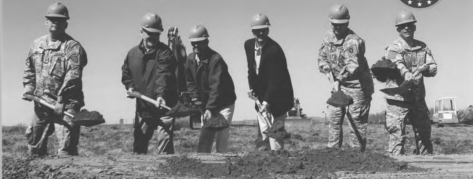
New Bethel Readiness Center Begins. The official party digs up dirt as a sign of “breaking ground” for the start of construction of the new Bethel Readiness Center. So far, the contractor has poured the concrete, insulated side panels and put roof panels in place. The project is ahead of schedule and is expected to be completed by December 2011. From left: Brigadier General J. Randy Banez, assistant adjutant general, Alaska Army National Guard; Representative Bob Herron, Alaska State Legislature; Jim Miller, project superintendent, Unit Construction; Lieutenant Governor Craig Campbell; First Lieutenant Jason Caldwell, commander, B Company, 1/143rd Infantry Regiment, Alaska Army National Guard; Major General Thomas H. Kalkus, adjutant general, Alaska National Guard. Photo: Private First Class Karina Paroan, DMVA Public Affairs.
