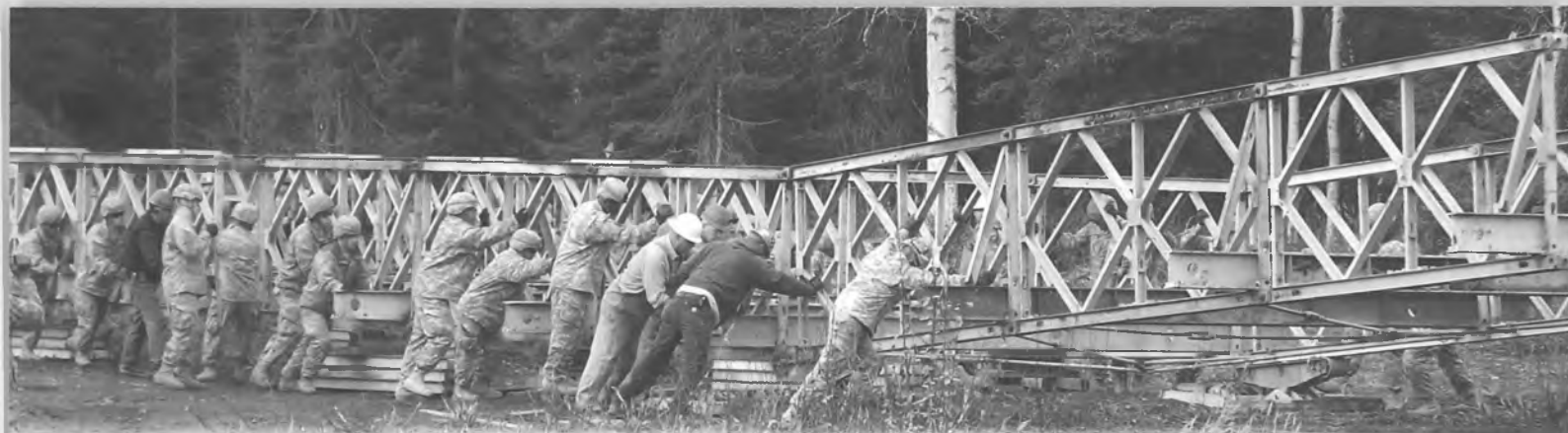
Building Bridges and Partnerships. State Department of Transportation workers and active-duty Army Soldiers construct a temporary bridge. Photo: Meadow Bailey, Department of Transportation
