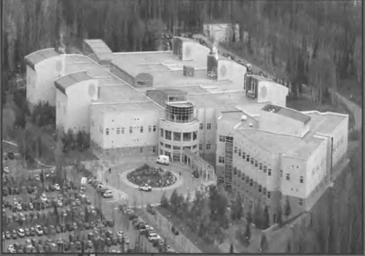
VA/DOD Joint Venture Hospital Joint Base Elmendorf-Richardson
