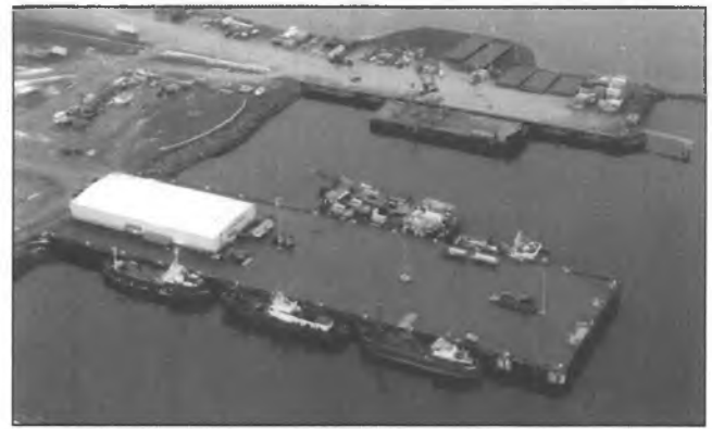
ARRC's West (left) and East docks in Seward.
