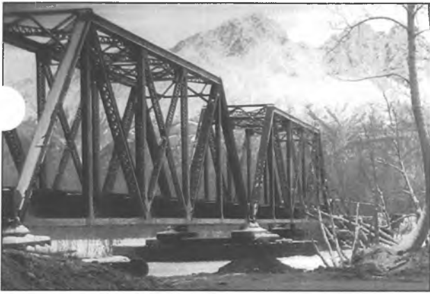
Matanuska River Bridge is undergoing rehabilitation work.
