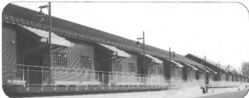
RENOVATING THE HISTORIC FREIGHT SHED TO LEADERSHIP ENERGY & ENVIRONMENTAL DESIGN (LEED) STANDARDS IS A MAJOR INTERNALLY-FUNDED PROJECT.
