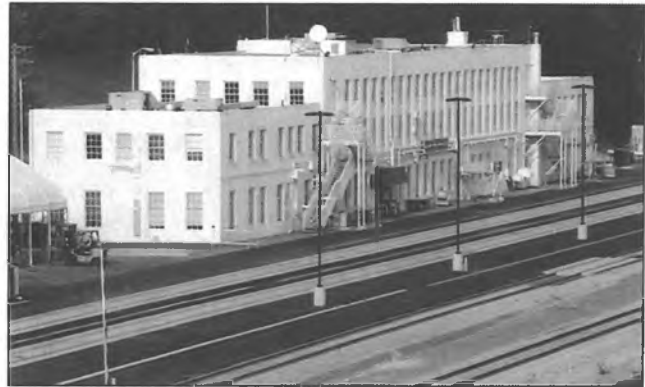
Phase One of the Ship Creek ITC constructs two new tracks and a pedestrian platform next to the Anchorage Historic Depot.
