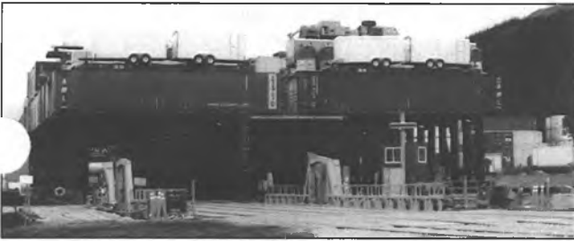
The Whittier barge slip stern (front) is replaced. The towers were removed and replaced by hydraulic devices to lower/raise the slip.
