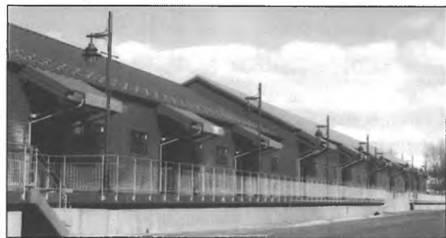
The Historic Freight Shed renovation nears completion.
