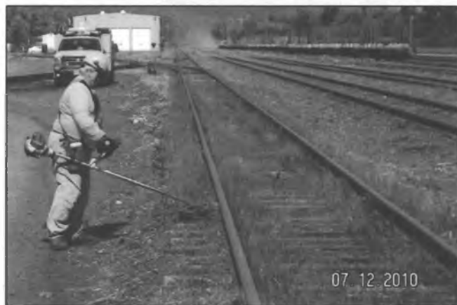
Ineffective mechanical/manual control in Seward yard prior to herbicide application.
