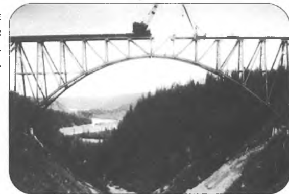
HURRICANE BRIDGE UNDER CONSTRUCTION. CIRCA 1921.
