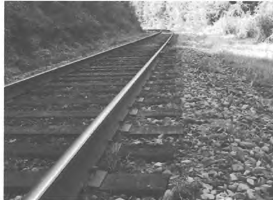
The herbicide works effectively on weeds between the ties, without migrating or lingering in the soil.
