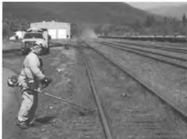
A Railroad track maintenance worker manually controls weeds in the Seward yard. Herbicides are far more effective for controlling vegetation within the rail yards.
