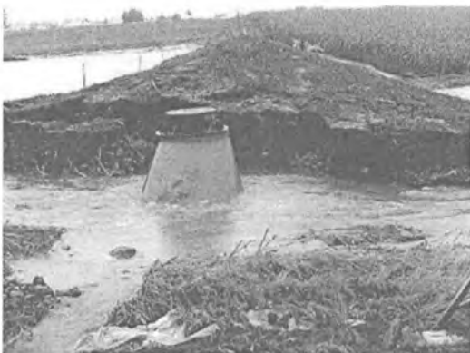
Storm sewer overflow following a precipitation event.
