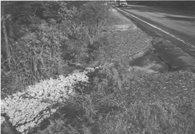
Curb-less roadside, equipped with stormwater drainage system in Cohasset, Mass.
