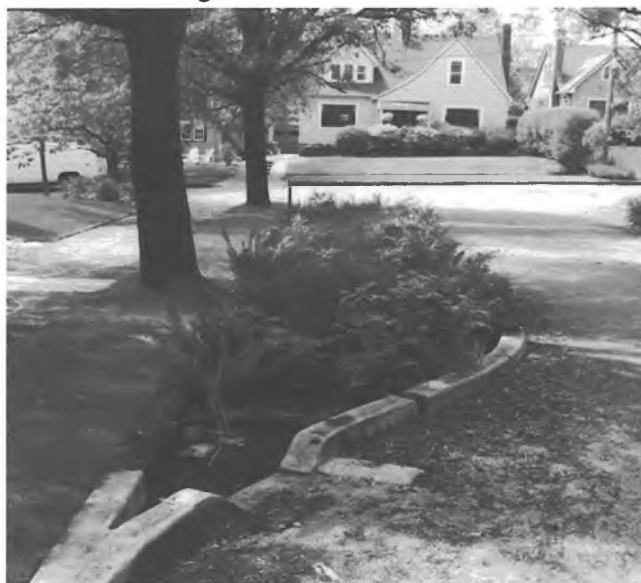
Vegetated swales capture and infiltrate runoff along this "green street" in Portland, Oregon.
