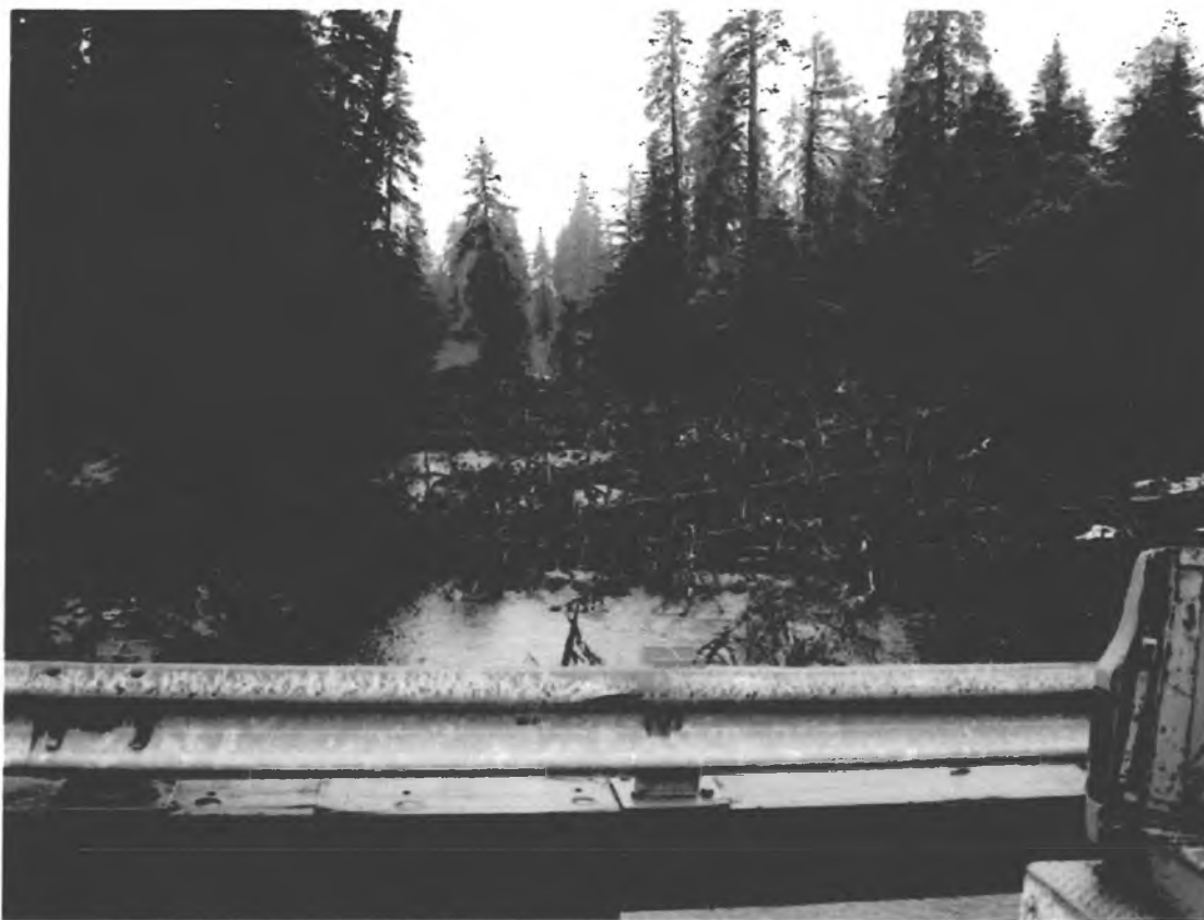
Figure 4 Failed riparian buffer West Fork of the Situk River
