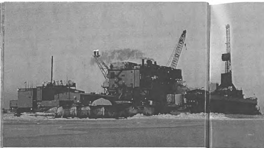
Northstar's production facilities were built in Alaska and sea lifted to the North Slope.
