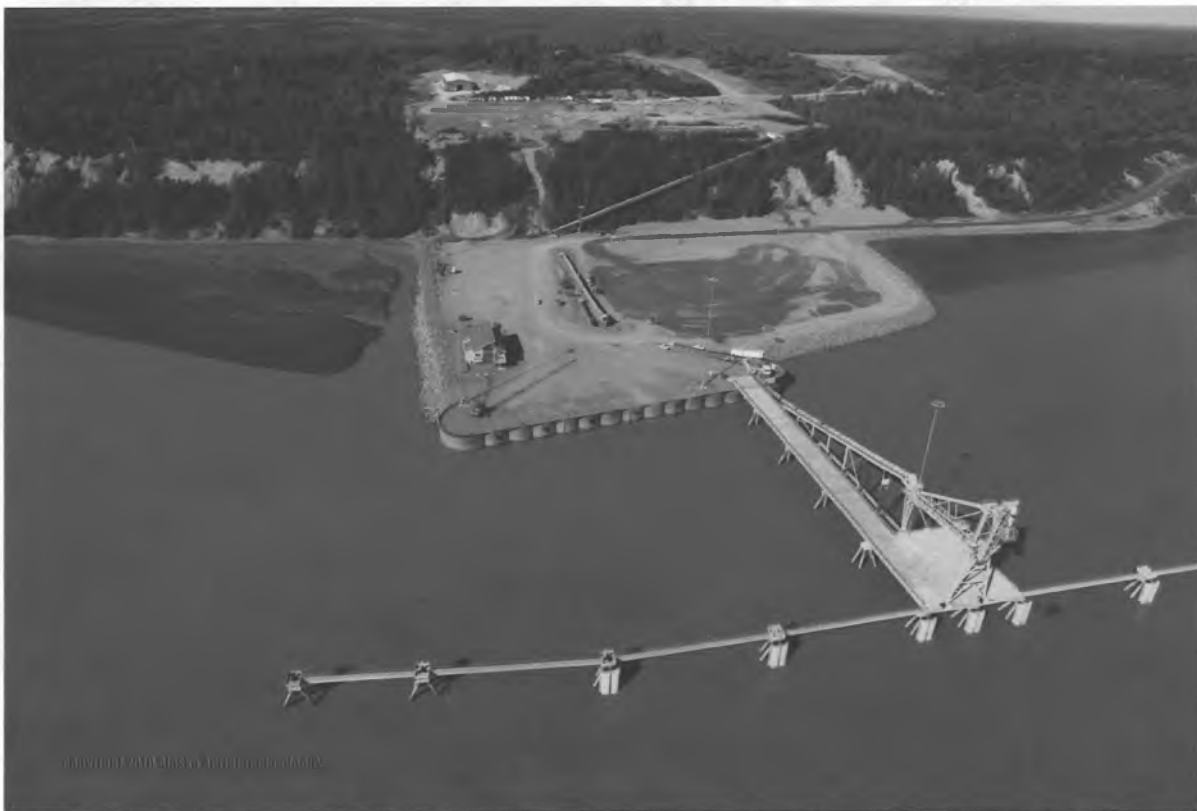
Figure 7-7: Port MacKenzie (Photo courtesy of Port MacKenzie and Alaska Aerial Technologies)
