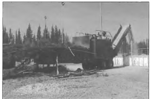
The Rotochopper processing whole trees and depositing the woodchips into the school’s hockey rink for storage. Photo: DOF
