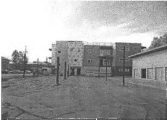
Photograph of Property (construction underway):
