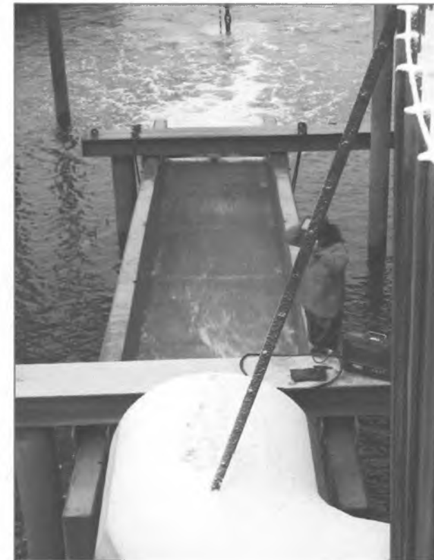
Fish ladder after construction
