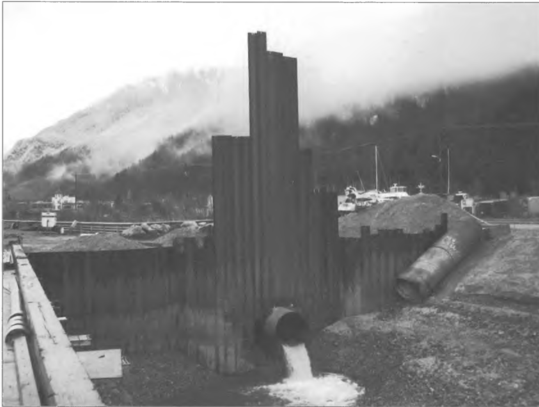
OPEN CELL bulkhead under construction with culvert penetration
