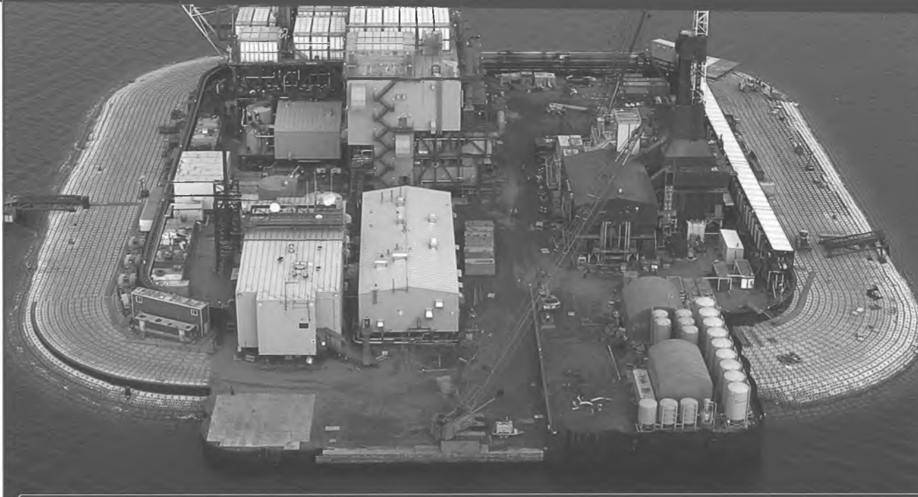
NORTHSTAR ISLAND BEAUFORT SEA, ALASKA BP Exploration (Alaska), Inc.
