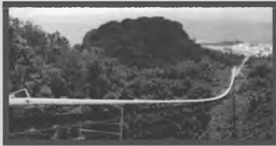
Elevated coal conveyer to reduce environmental impact
