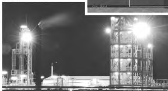
Chinchilla demonstration production facility
