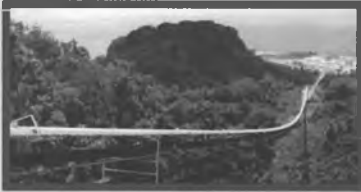
Elevated coal conveyer to reduce environmental impact
