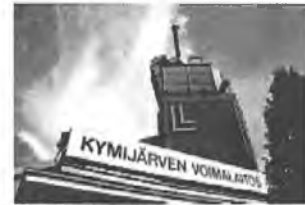
Construction of the new power plant. Photos: Nina Näsman
