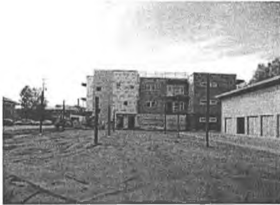
Photograph of Property (construction underway):
