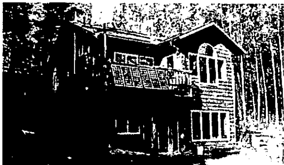
Home near Fairbanks that uses a combination of photovoltaic cells for power, an active solar water heater, and passive solar design.
