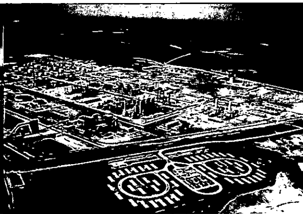
South African Mossgas 47,000 BPD Gas to Liquids (GTL)
