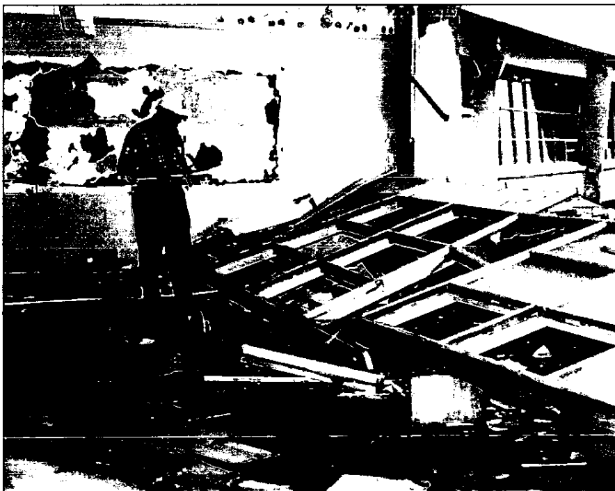
Figure 4. Anchorage High School, 1964 Alaska earthquake (photo credit Anchorage Museum).
