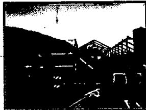
Construction began in late FY07 to increase capacity at the ARCH residential treatment facility in Eagle River.
