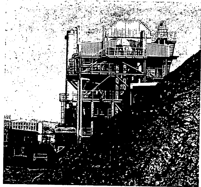
2 MW plant in Güssing, Austria
