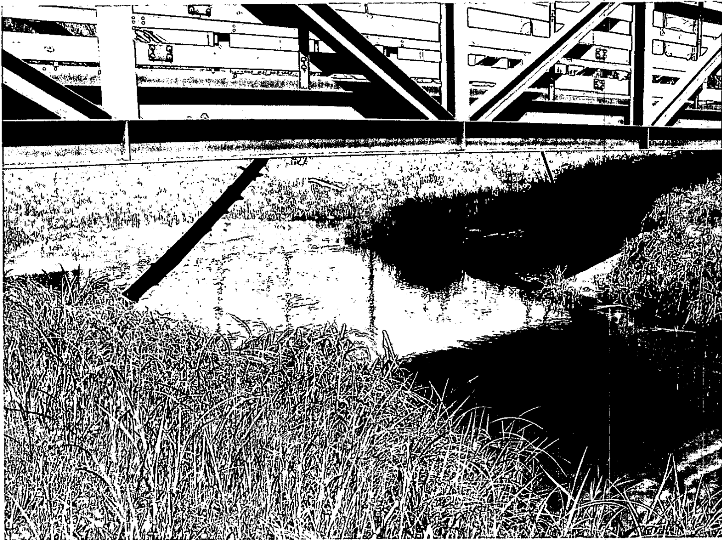
Multi-use trail bridge, Tidewater Slough, Girdwood , Alaska
