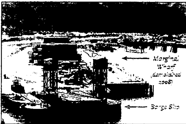
The barge slip and marginal wharf in Whittier.
